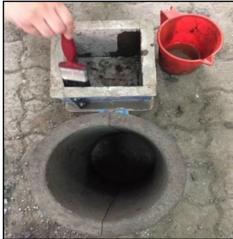
Fig-6: Applying oil to the moulds (Source: CCE ML)
