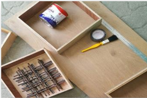
Fig-2: Slab moulds & steel rebar
