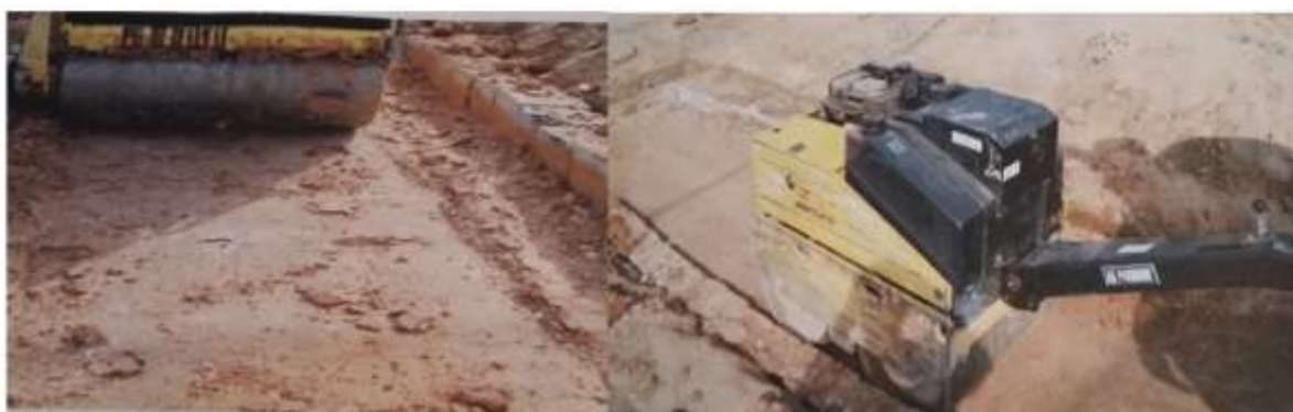
Fig-1: Field compaction test – field model
