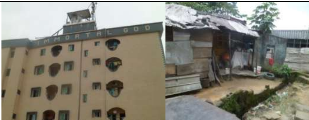
Fig-3: Substandard and Standard buildings identified in some urban Fronts of Douala
