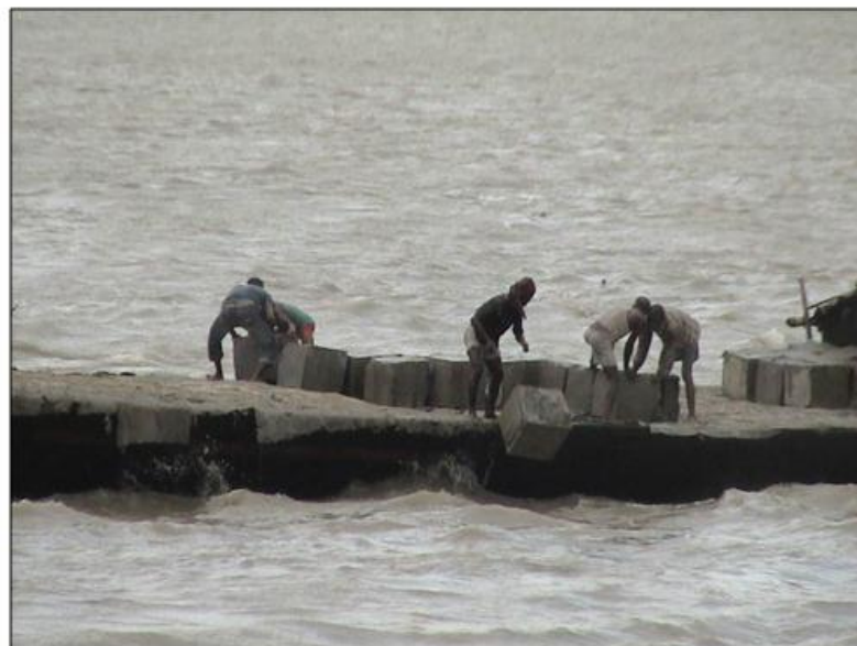
Photograph-1: CC blocks are being dumped for toe protection in the Jamuna River at Sirajgonj Hard Point, Shirajganj, Bangladesh
