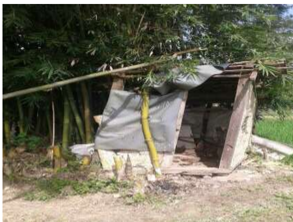
Photo-7: A typical human toilet in Son La province
