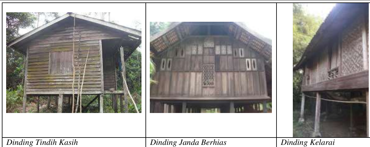
Fig-8: Wall as part of the architectural elements in traditional Malay house system [19]
