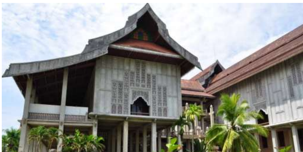
Fig-11: Example of concrete wall with traditional aesthetic elements applied at Terengganu State Museum
